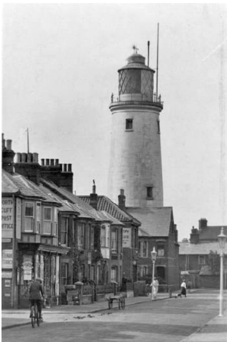
Stradbroke Road and the Lighthouse in 1930s. It was built in 1887 and the light is 37 m above mean high water. It was automated and electrified in 1938. Southwold Museum P1723
