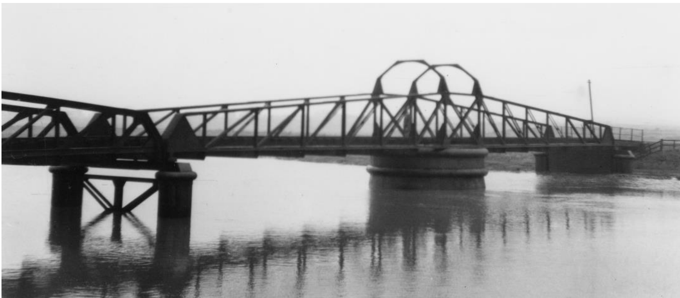
The River Blyth presented the major civil engineering challenge for the Railway. The bridge featured a pivoting span to allow boats to pass. This photo shows the bridge after it had been adapted in 1907 to make it compatible with standard-gauge rolling stock in anticipation of compulsory standardisation which never actually took place. Photo by Ronald Shepherd. Copyright West Sussex County Council Record Office. Southwold Museum P2416
